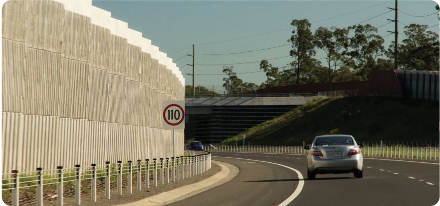
Unbroken edge line.
